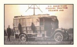
During the early 1900s, the Army operated from mobile as well as fixed installations. The museum displays a picture of a mobile U.S. direction finding truck, or "tractor" in the terminology of the time. The truck had a DF antenna, which was turned by hand from the inside. By measuring the angle of entry and the skip of a signal coming in and bouncing off the ionos-
