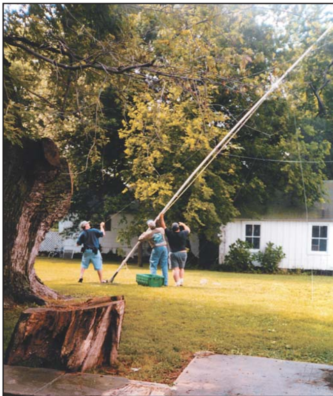
The antenna mast goes up in preparation for the start of the Smith Island operation.
